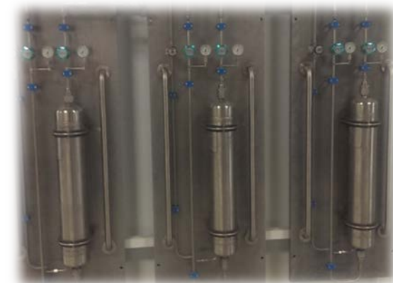
Three (3) NANOCHEM® MAX™ purifiers each capable of purifying 3000 slpm (180 m3/h)
